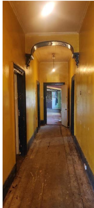
Main hallway (main building)
