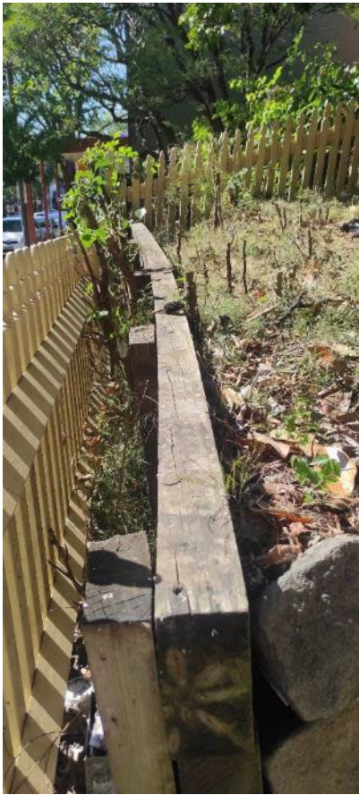
Existing retaining wall
